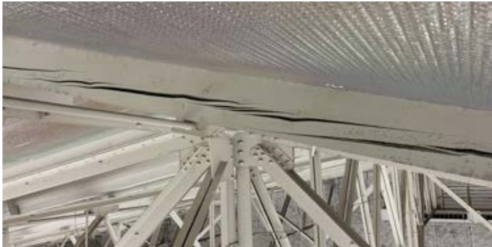
TMC – Structural Repairs
