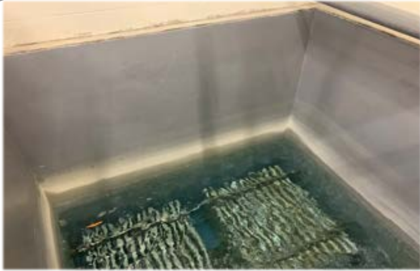
TALC – Filter Tank Repair
