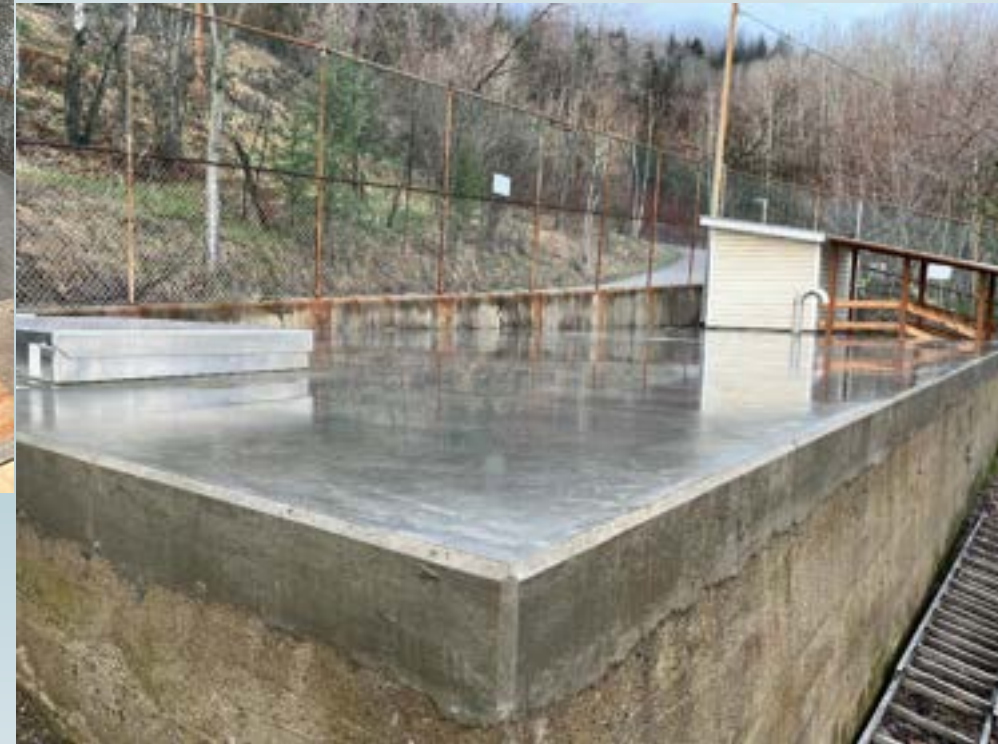
Lookout reservoir – New roof
