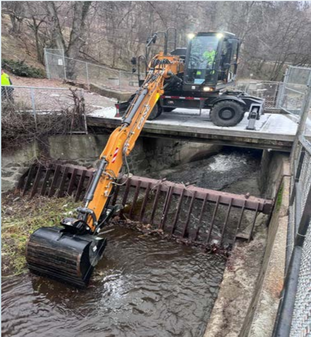
New Wheeled Excavator
